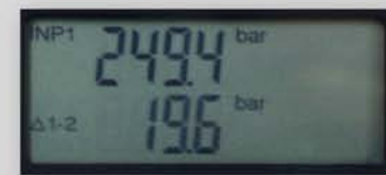
Screen shot showing differential pressure
